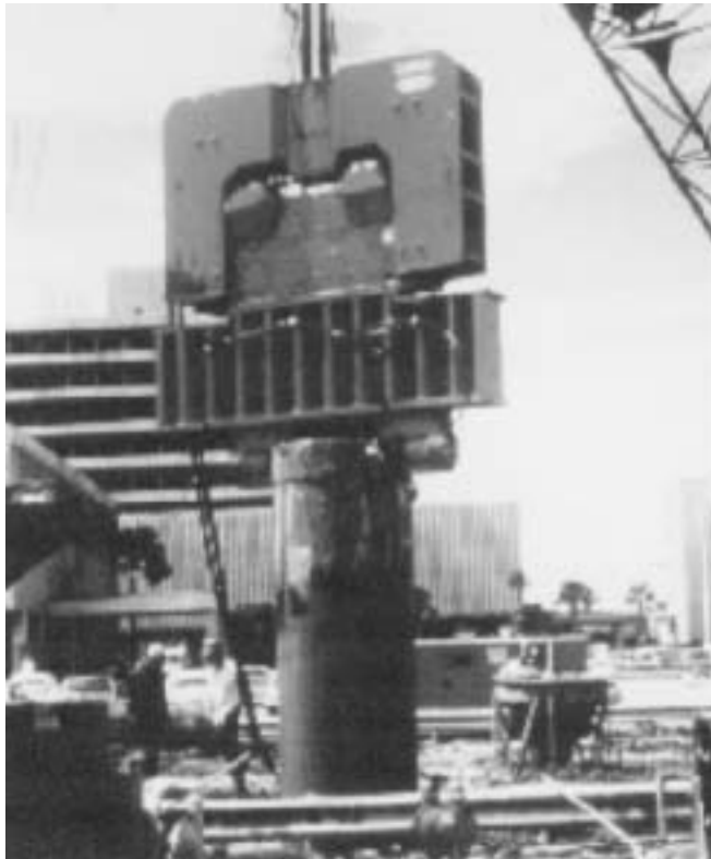
Figure 14.7 Vibratory pile driver (Courtesy of Michael W. O'Neill, University of Houston, Texas)
