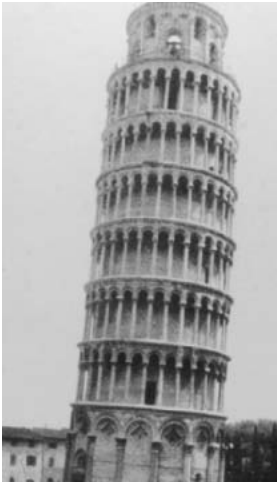
Figure 1.1 Leaning Tower of Pisa, Italy (Courtesy of Braja Das)
