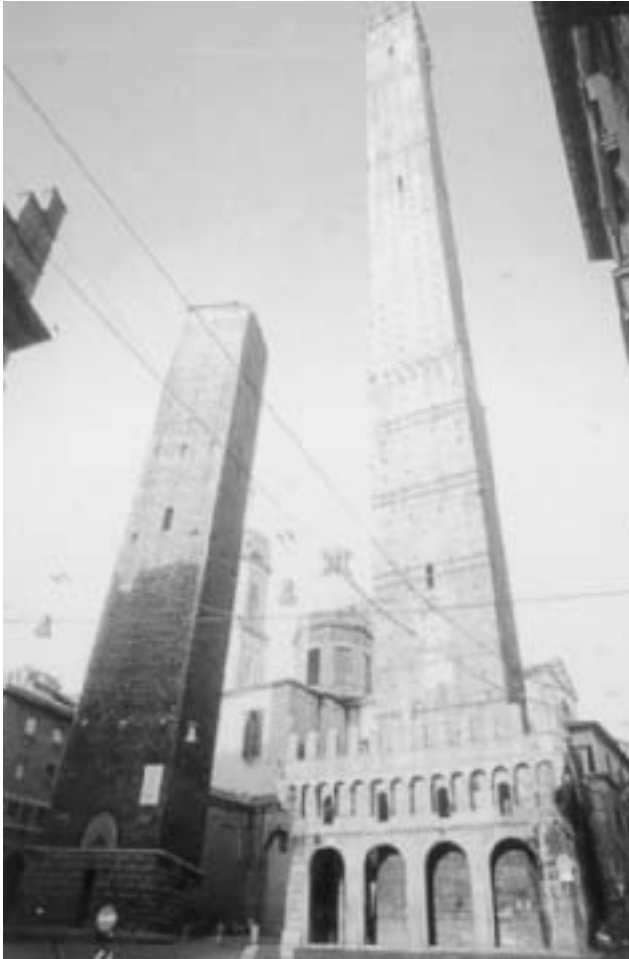
Figure 1.2 Tilting of Garisenda Tower (left) and Asinelli Tower (right) in Bologna, Italy (Courtesy of Braja Das)
