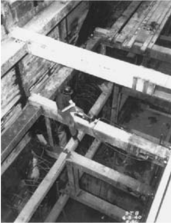
Figure 13.19 Braced cut in Chicago subway construction (Courtesy of Ralph B. Peck)
