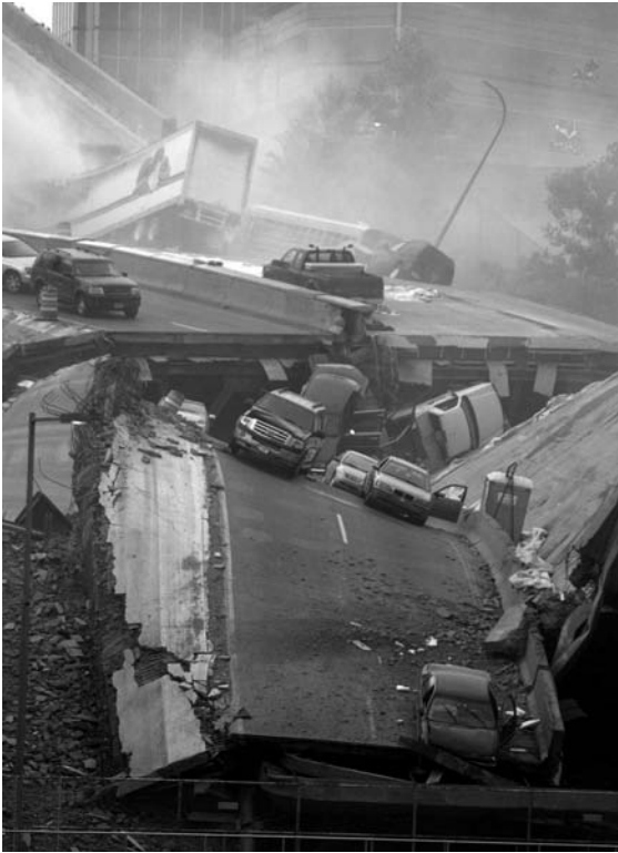
Interstate 35W Bridge Collapse in Minnesota (2007)
