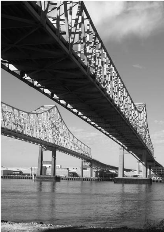
Truss Bridges Terry Poche/Shutterstock
