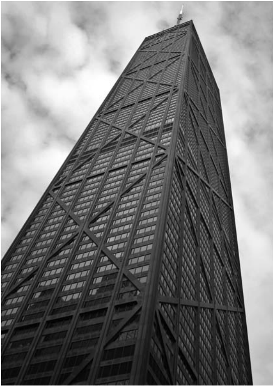
The John Hancock Building, Chicago
