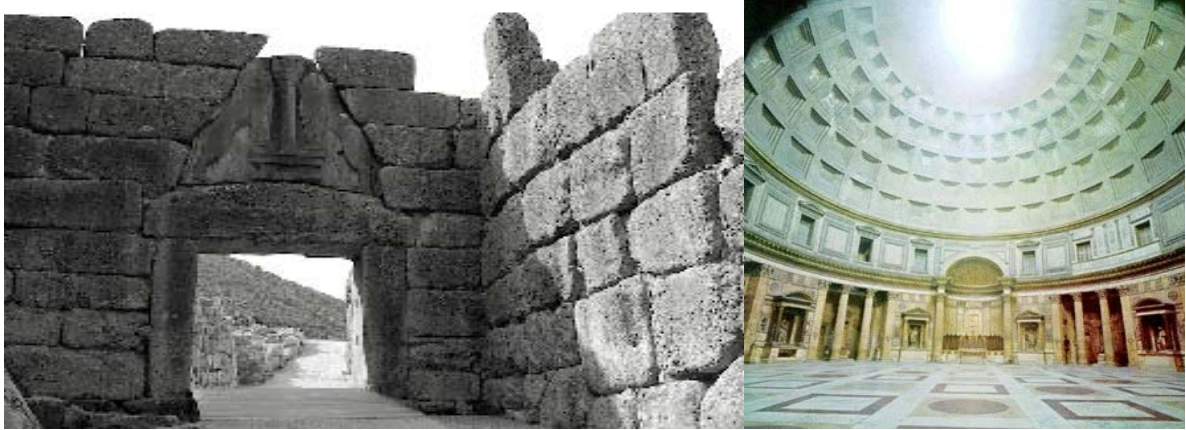
Figure 2: Lion Gate in Greece: Stone gate constructed in 1350 B.C. and the Agrippa's pantheon in Rome: Temple of all the gods made of unreinforced concrete with pozzuolana.
