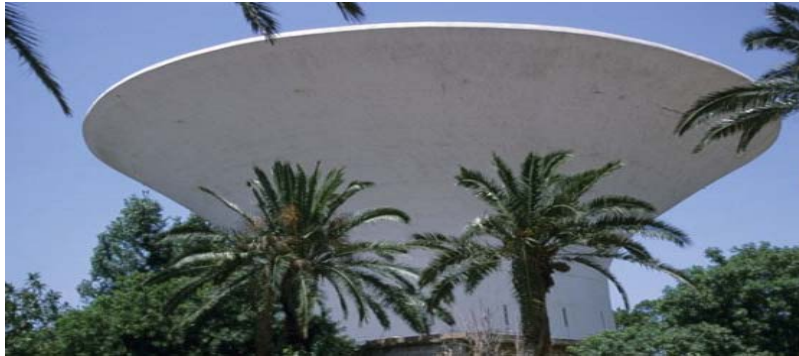
Figure 6: Fedala water tank : hyperbolical-concrete silo for the storage of water in Morocco.
