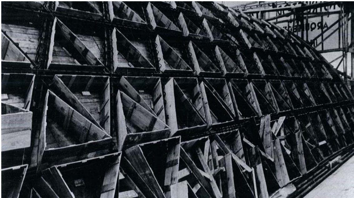
Figure 69: Construction of the skylight beams using wooden frameworks.
