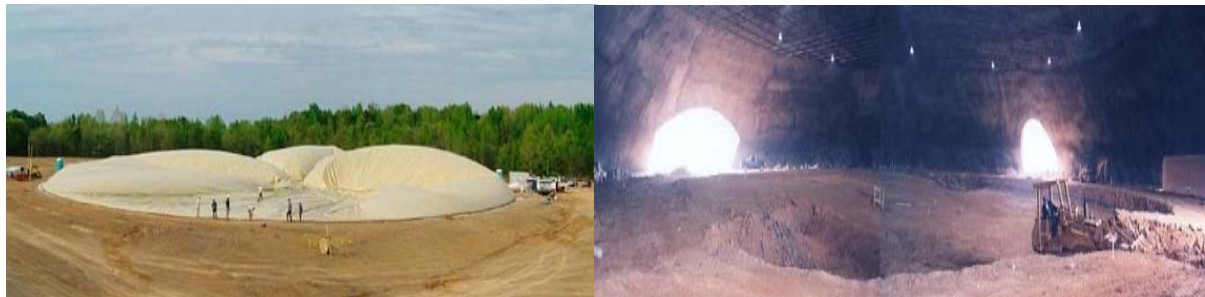
Figure 16: Inflating process using polyurethane foam and Application of the shotconcrete.
