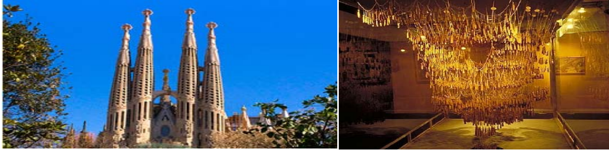
Figure 5: Sagrada Família in Barcelona and Antonio Gaudí's reversed model used to determine the forces in pure compression.
