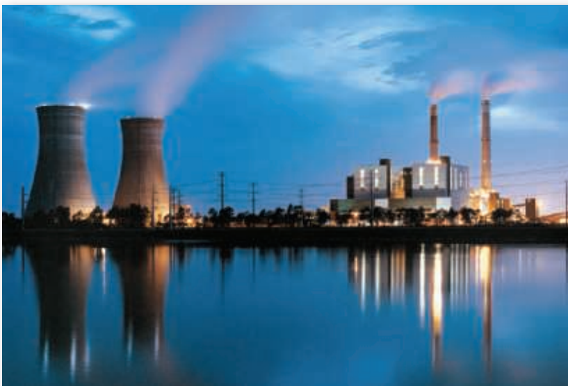
Orlando Utilities Commission
