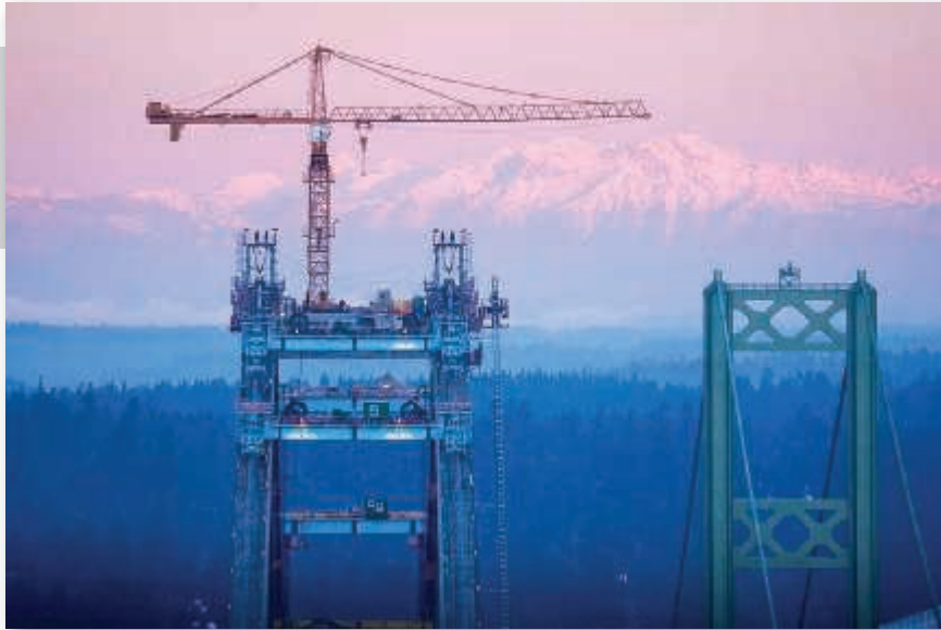
Courtesy of Bechtel Corporation
